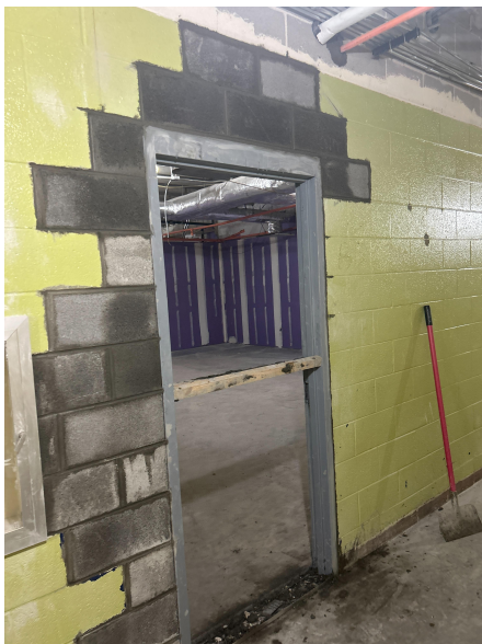
Installing CMU and door frames on level 1.
