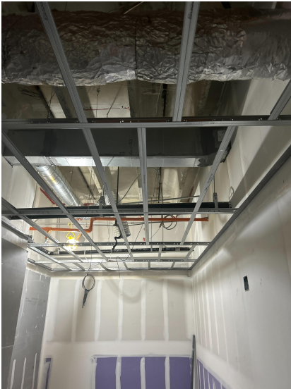
Installing ceiling grids in restrooms on level 2.
